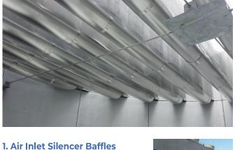
Made of sea water resistance aluminum - could be delivered with tailored casing.
