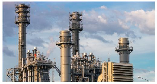
H+R Flue Gas Silencers, which are usually behind the turbine, are well suited for very high temperatures (up to 720°C) in combination with high flow velocities.
